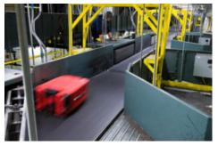
ELS has provided the operations and maintenance services for the Hartsfield-Jackson Atlanta International Airport North Terminal since the middle of the last decade. The BHS has more than 15,000 feet of conveyor and 800 electric motors (480 volt, three phase) ranging in size from 2 to 7% horsepower.
